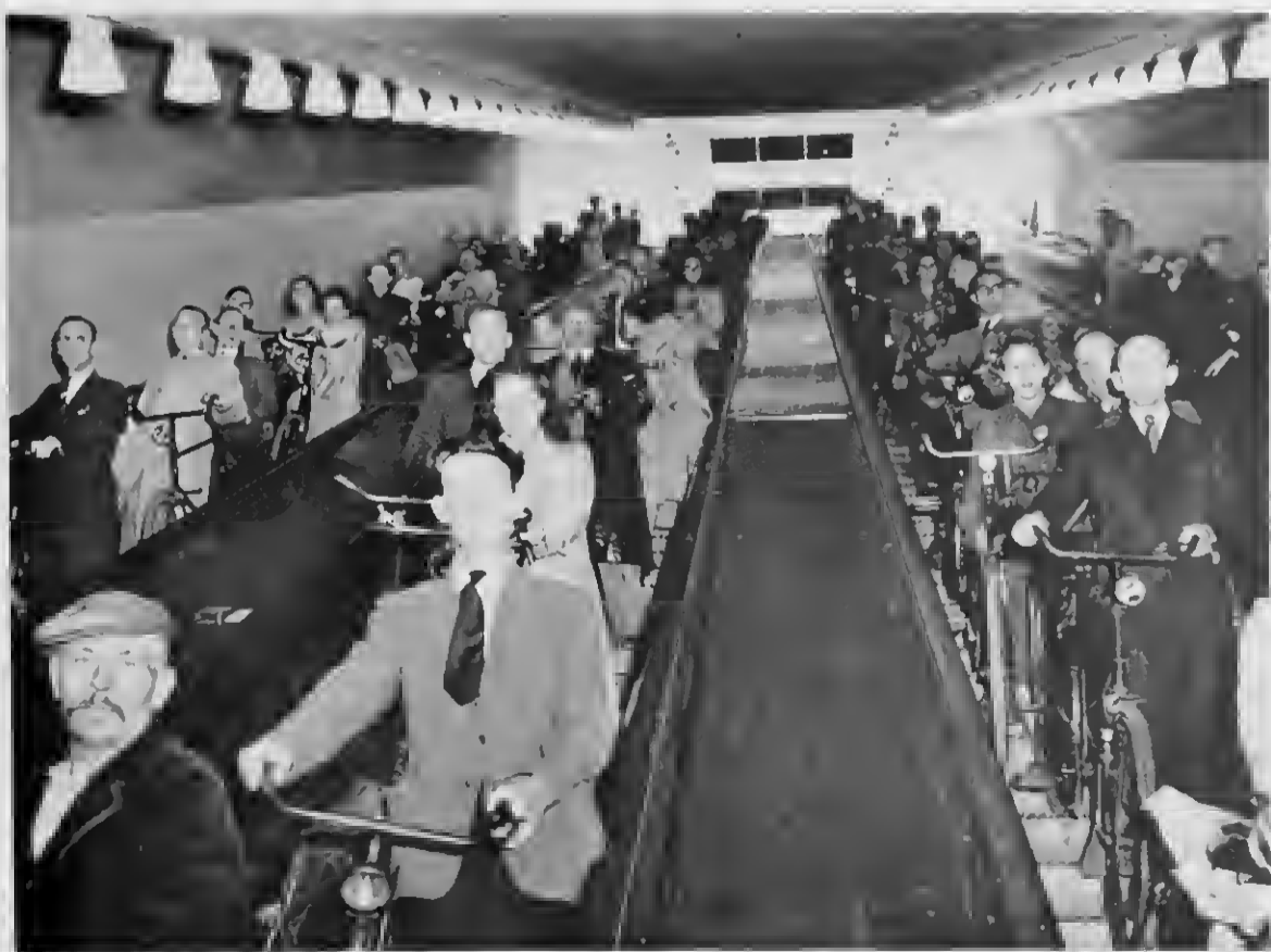
This escalator in the Maas Tunnel in Rotterdam was built especially for cyclists and their vehicles. Here it is in use during rush hour, carrying a full load.
